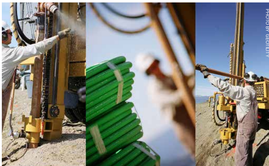
Installing a ground heat exchanger for a GeoTility project in Kelowna, B.C.
